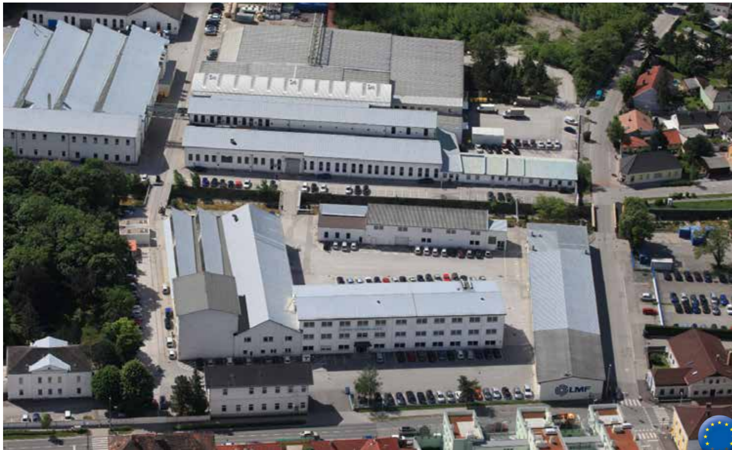
LMF headquarters in Leobersdorf, Austria.
